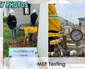
Witness of water leak test
